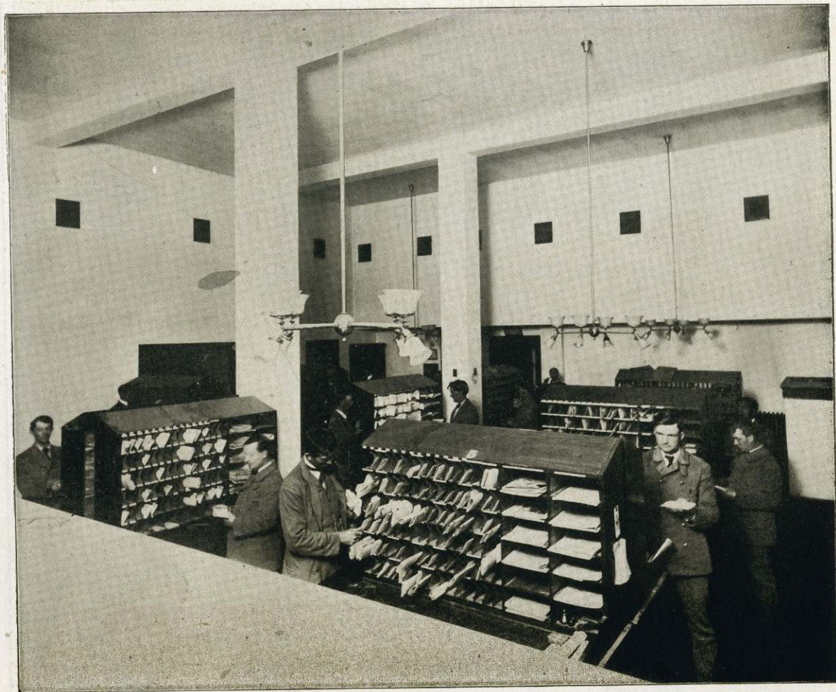
City and Rural Letter Carriers' Work Room, 1216 Square Feet.
