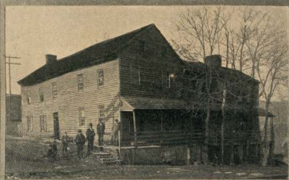
Old Post Printing Office—the Oldest Printery West of the Alleghenies, Established 1803. A Fourteen-foot Fire Place, Carrico Building, Stood on Present Site I. O. O. F. Temple. Old Franklin Hotel, Erected 1774—torn down 1895—site, present Franklin Hotel.
