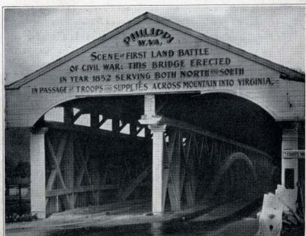
COVERED BRIDGE AT PHILIPPI
