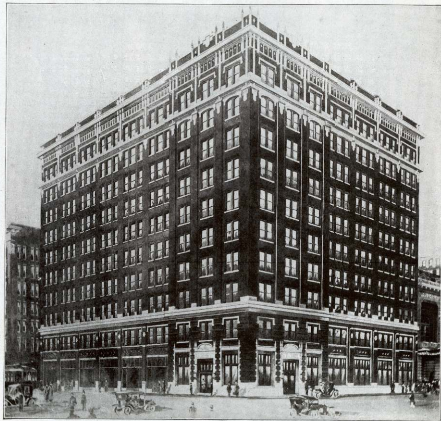
Miller-Ritter Office Building
