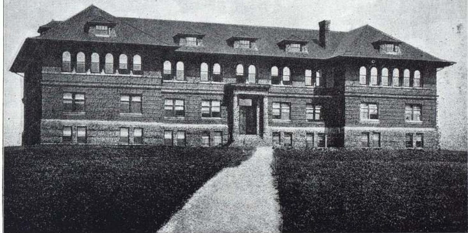
AGRICULTURAL BUILDING, PENNSYLVANIA STATE COLLEGE. Another View to Show that Our Neighbors Believe in Scientific Agriculture.
