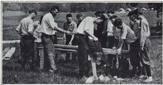
WORK , if it's interesting, is just about as good as play. These boys are on the level about trying to learn some of the principles of carpentry.
