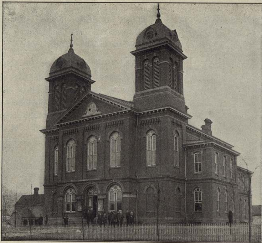
MARSHALL COUNTY COURT HOUSE.
