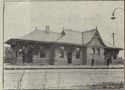
OHIO RIVER RAILROAD DEPOT
